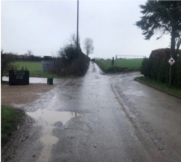
Short Street towards Station Road.
