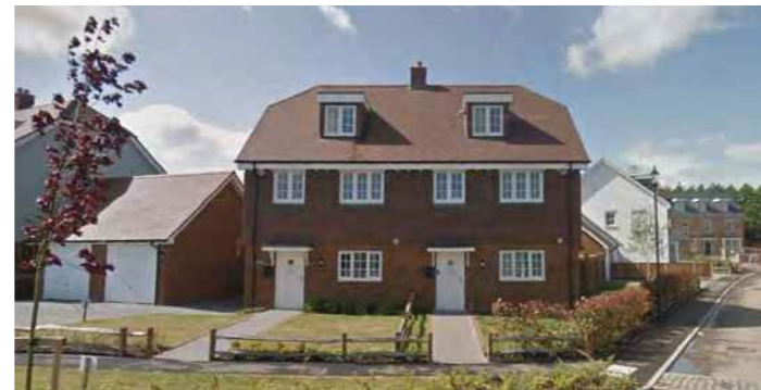
Red Brick, Rafter Feet, Barn Hipped Roof, Dormer Windows
