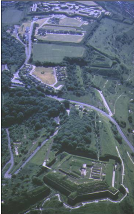
Aerial view of the Western Heights looking east to west (copyright KCC)
