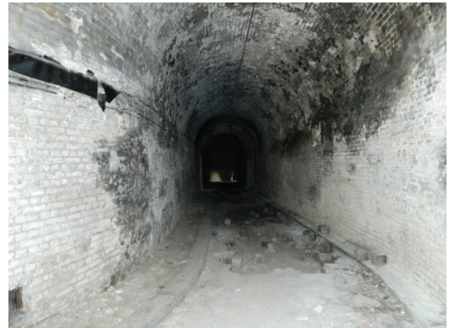
The North Entrance Tunnel
