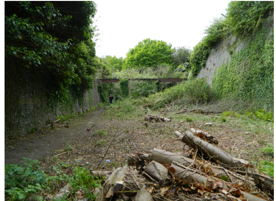
Subterranean defensive works that lie beneath the colonising mantle of invading vegetation
