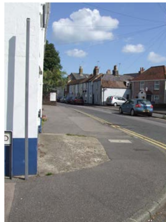
Pavement tarmacked in West Street
