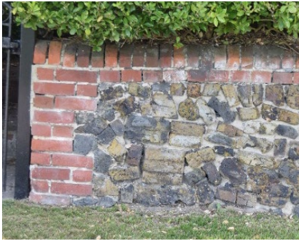
Burr brick walls on Hotel Rd.
