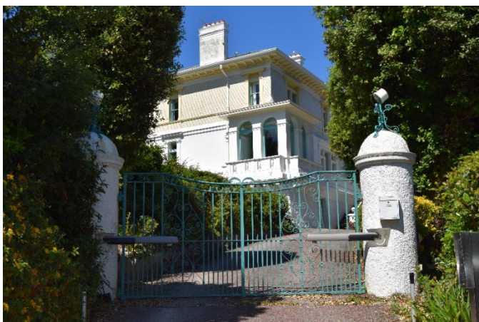
South Foreland House
