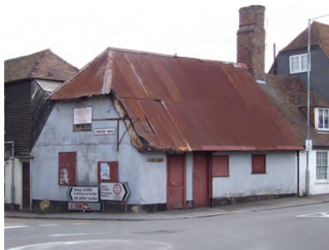
Listed Building in poor repair
