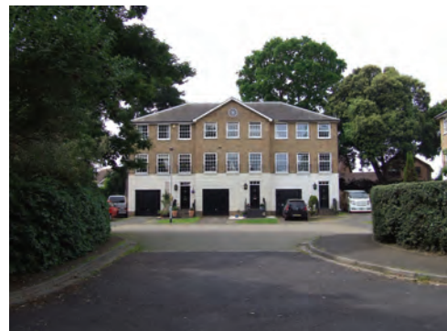
Modern development showing use of materials prevalent in the conservation area, brick and render.
