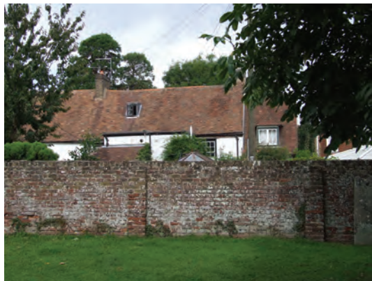
Kent peg tiled roof on a historic building
