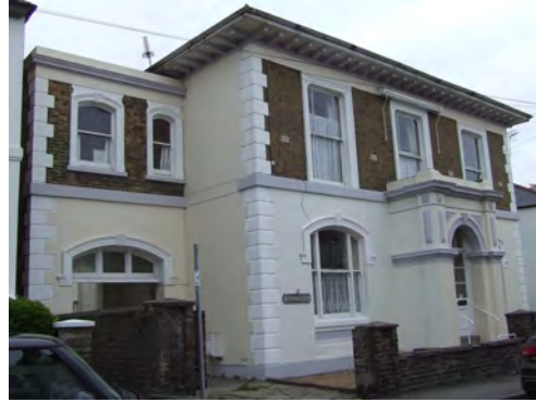
Victoria Lodge, with its deep overhanging eaves and prominent porch
