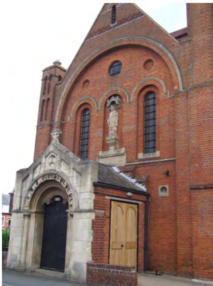
The dominant red brick facade of Church of Saint Thomas
