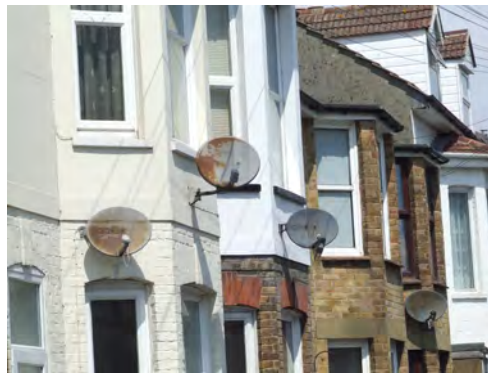
Satellite dishes scattered across the front elevations of buildings
