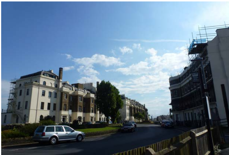
Looking towards the 60th Rifle Memorial and the rear of Waterloo Mansions
