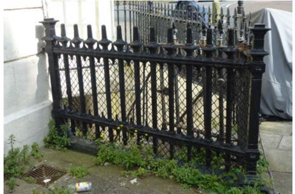
Remnant of railings to New Bridge House
