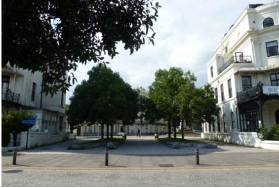
Well designed and detailed public realm works
