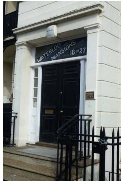
Entrance door to Waterloo Mansions
