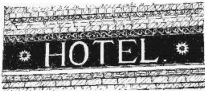
FIG. 19. Sign painting direct to a rendered wall-face framed in moulded brick.
