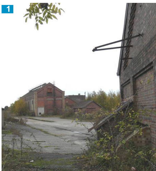
1. Derelict colliery buildings at Snowdown.
