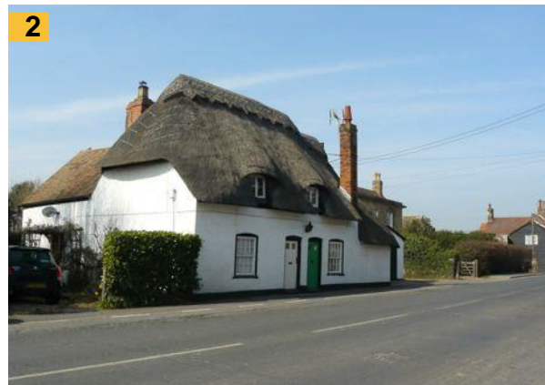
2. Grade II Listed early eighteenth century thatched cottages in Preston.
