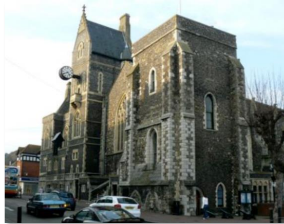
Figure 8.11 – Dover town hall – The Maison Dieu
