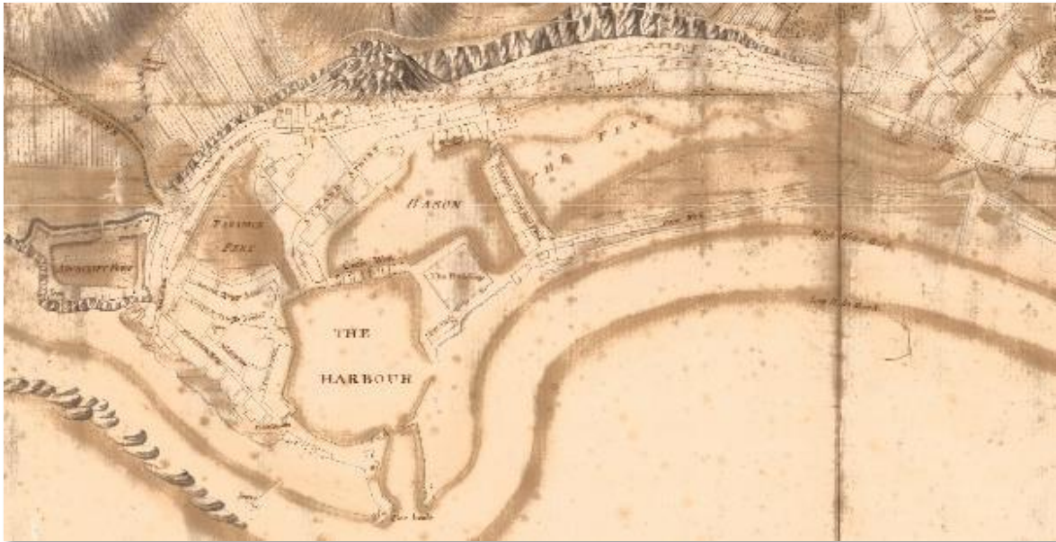
Figure 9.15 - Extract from Fouquet's 1737 map showing the 18 th century developments to the harbour
