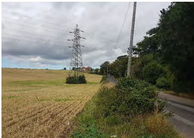
Arable fields south of Elvington, with large pylons interrupting the landscape
