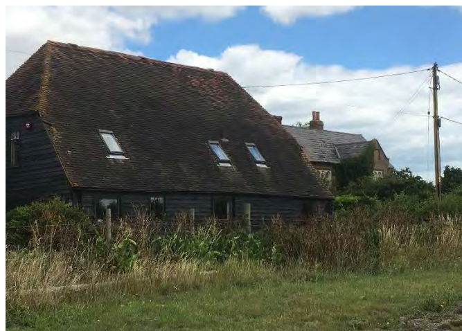
Black timbered farms are distinctive – now mainly converted for residential use
