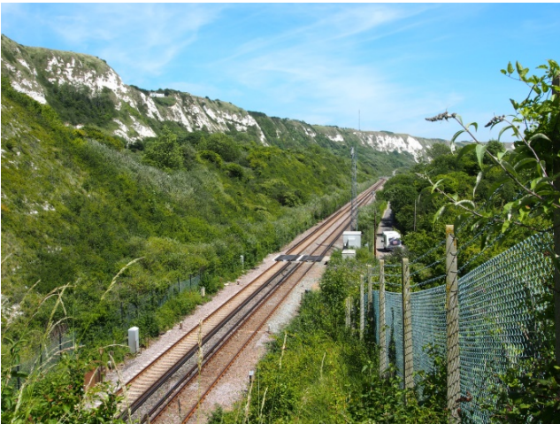
Landslips are not uncommon at The Warren, and the coastal railway line requires sea defences.
