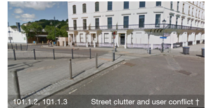
101.1.1 Lack of formal crossing †
