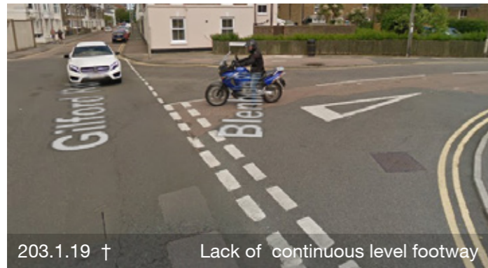
203.1.17 † Lack of continuous level footway
