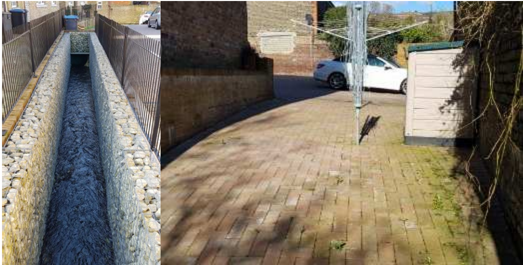
Figure 6 – Daylighted culvert at Lorne Road (left) and spillway connecting the carpark with the river (right).
