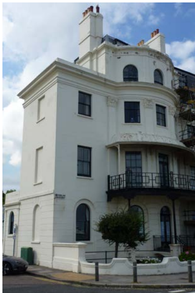
Corner house to Waterloo Mansions
