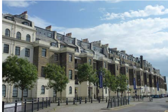
Waterloo Mansions - rear elevation
